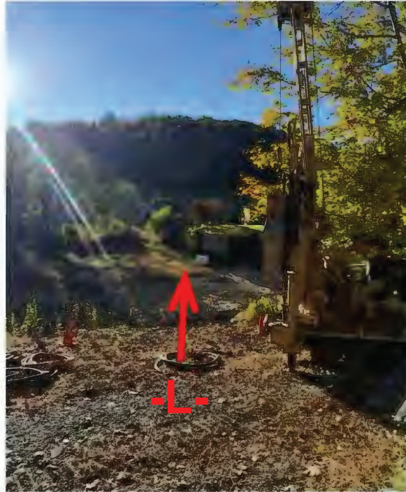
View Looking Upstation
